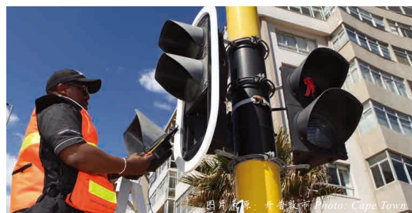
改造交通信号灯 Traffic lights being retrofitting
