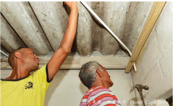
建筑屋顶翻新 Ceilings being retrofitted
