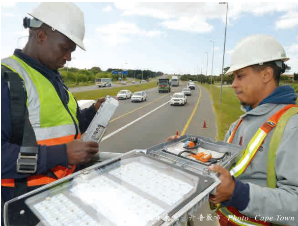
升级改造路灯 Retrofitting street lights
